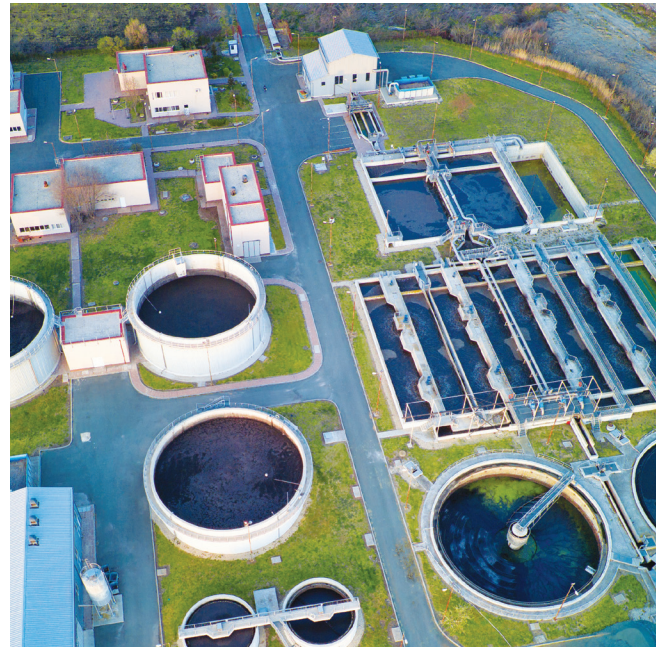
Sewage Water Treatment Plant
